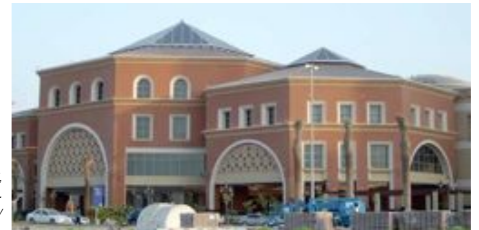
Mall of the Emirates in Dubai, United Arab Emirates. Precast supplied by United Precast Concrete.
