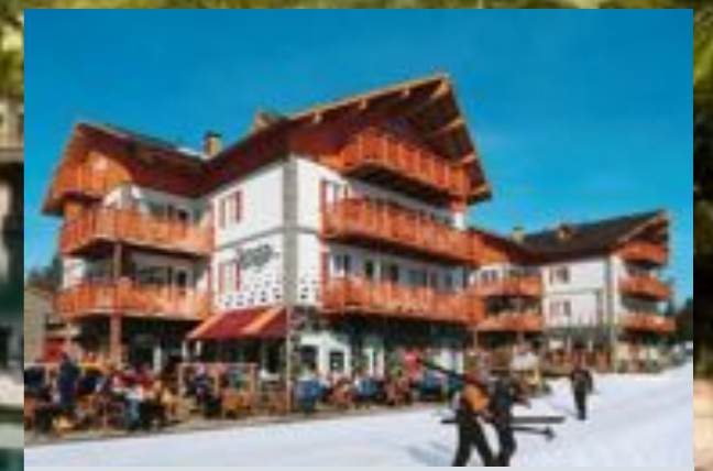
Levin Riekko, the holiday apartments with restaurant in Levi, Finland. Architect: Pertti Rantakokko. Full precast supplied by Ylitornion Betonituote YBT.
