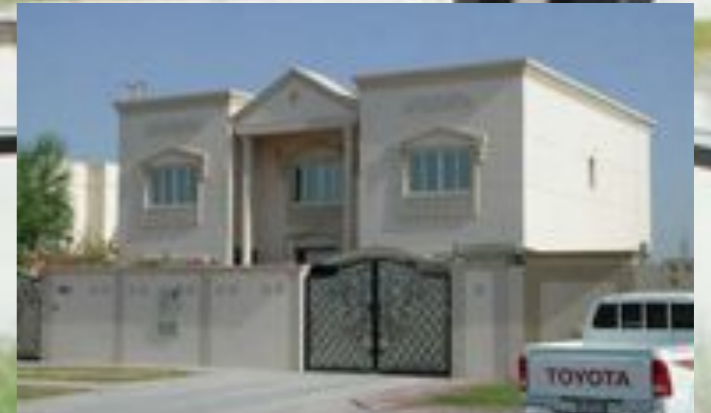
Low cost villa in Dubai, United Arab Emirates. Precast supplied by United Precast Concrete.
