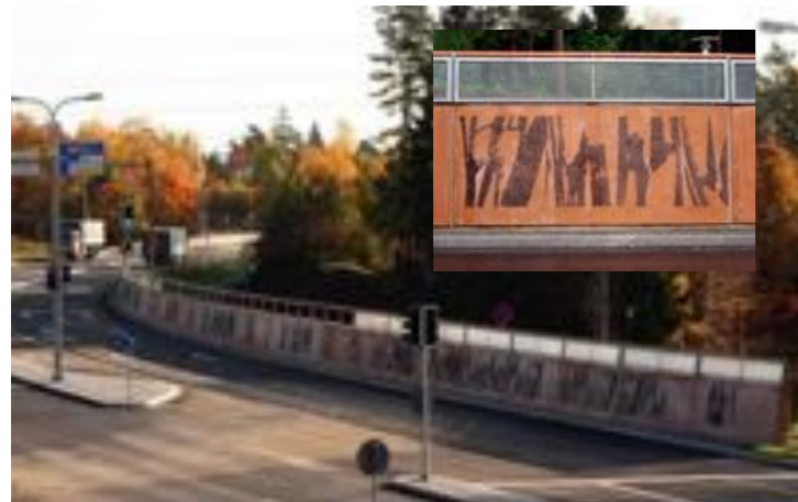
Sound barrier in Espoo, Finland. Architect: Ramboll Finland. Graphic Concrete™ Method for patterned concrete surfaces by Graphic Concrete Ltd. Precast supplied by Parma.
