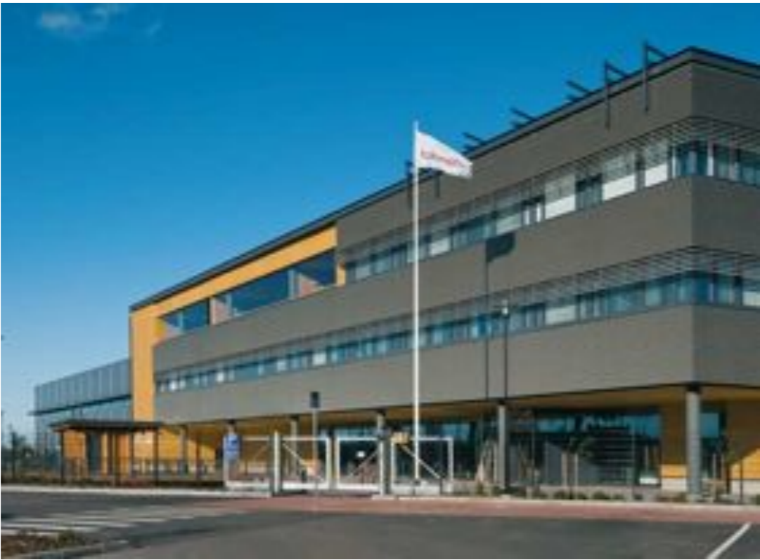
Logistics center in Mäntsälä, Finland. Architect: VG-Group. Builder: OKA. Full precast supplied by Parma.
