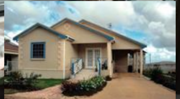
Affordable Income Housing Development in Cane Hill Terrace, St. Thomas, Barbados, West Indies. Builder: Spring Homes Limited. Precast supplied by Preconco Limited. Products used: floors, walls, columns, beams and stairs.
