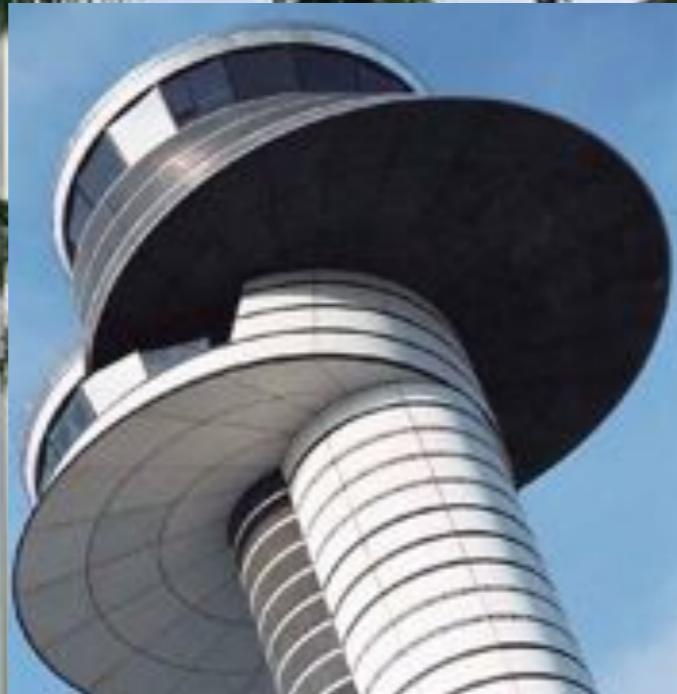
Control tower at Arlanda airport in Sweden. Architect: Wingårdh Arkitektkontor AB. Sandwich elements supplied by Strängbetong.
