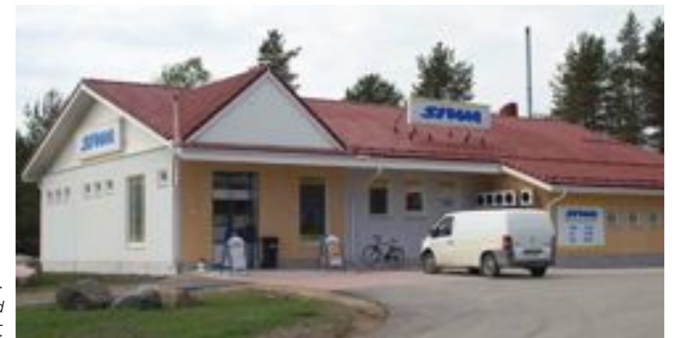
Siwa shop in Kemi, Finland. Full precast supplied and installed by Ylitornion Betonituote YBT.
