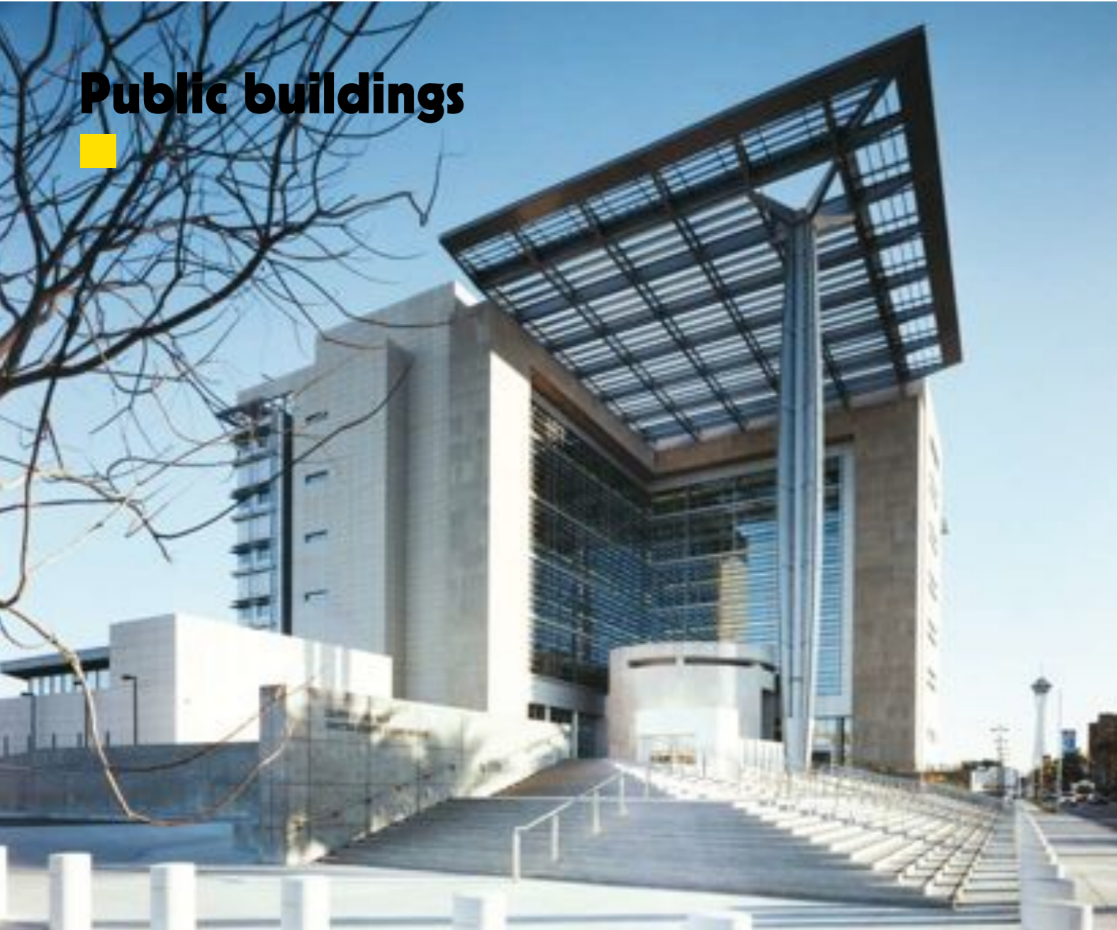
Lloyd D. George United States Courthouse in Las Vegas, USA. Architect: Dworsky Associates, Design Architect; Langdon Wilson Architects, Executive Architect. Precast supplied by Clark Pacific.
