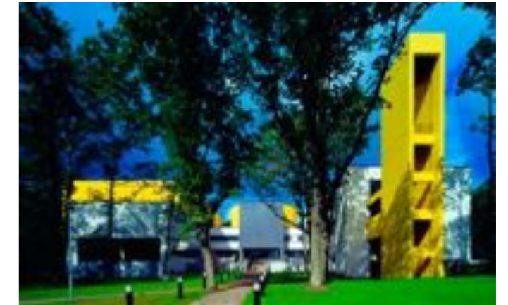
School in Rocca al Mare, Estonia. Architect: Ülo Peil, Architecture Office Urbel and Peil. Builder: KMG Ehitus AS. Precast supplied by E-Betoonelement.
