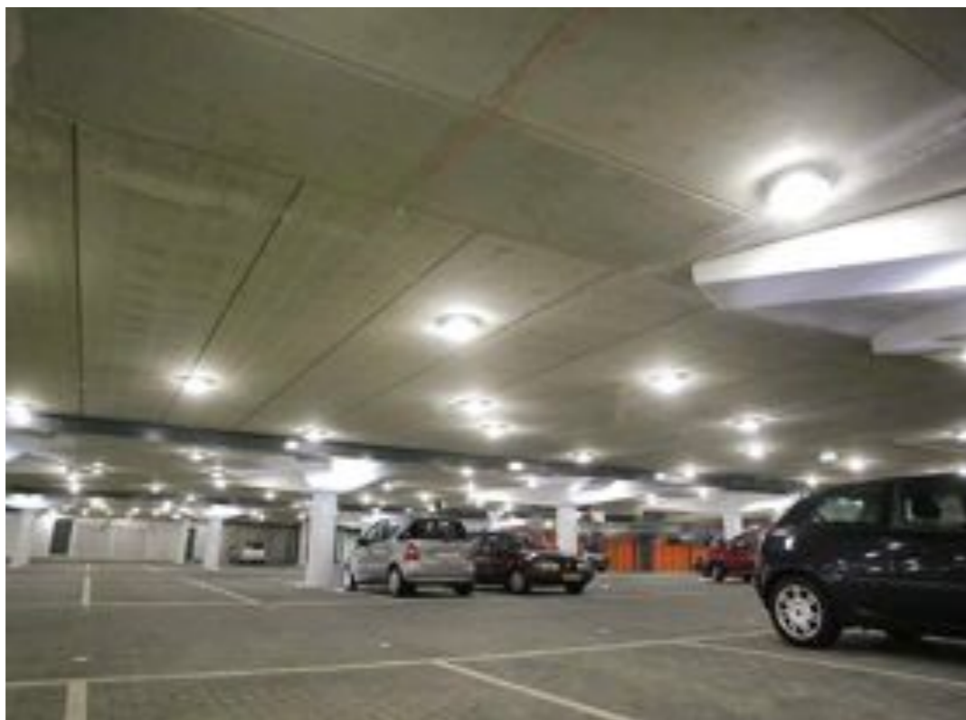
Car park in Heekplein, The Netherlands. Hollow-core slabs supplied by VBI.
