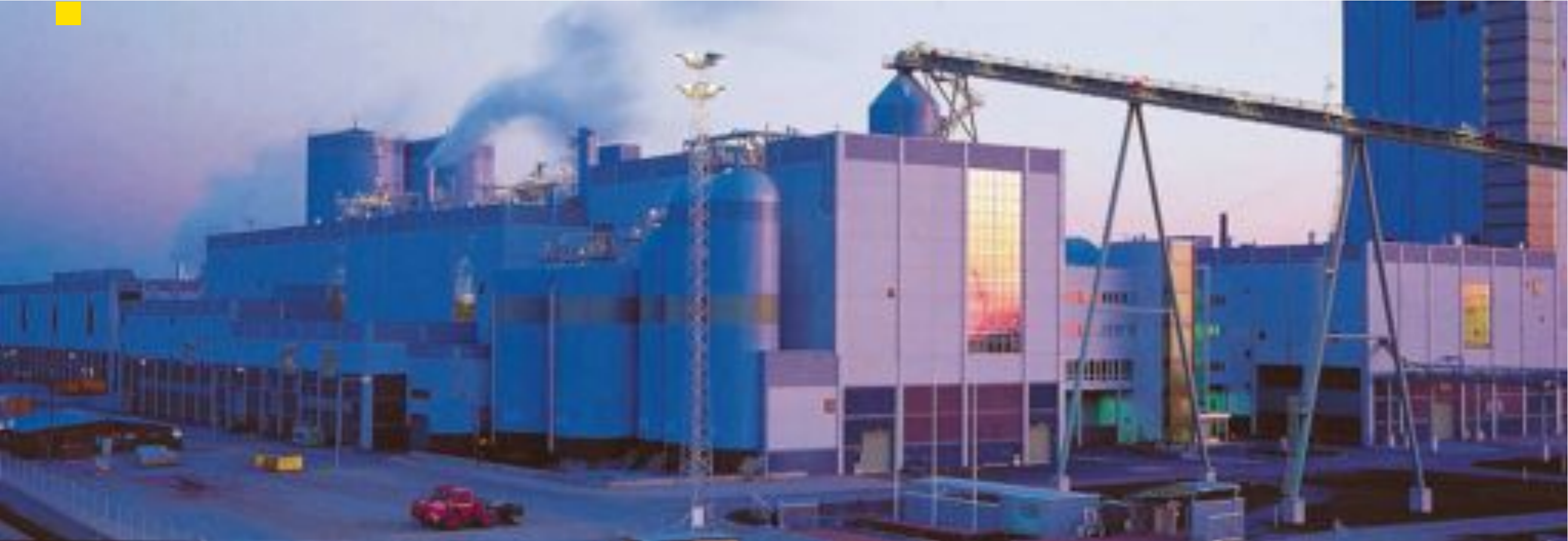
Pulp factory in Rauma, Finland. Architect: UKI-Arkkihtedit. Builder: Hartela. Full precast supplied by Parma.
