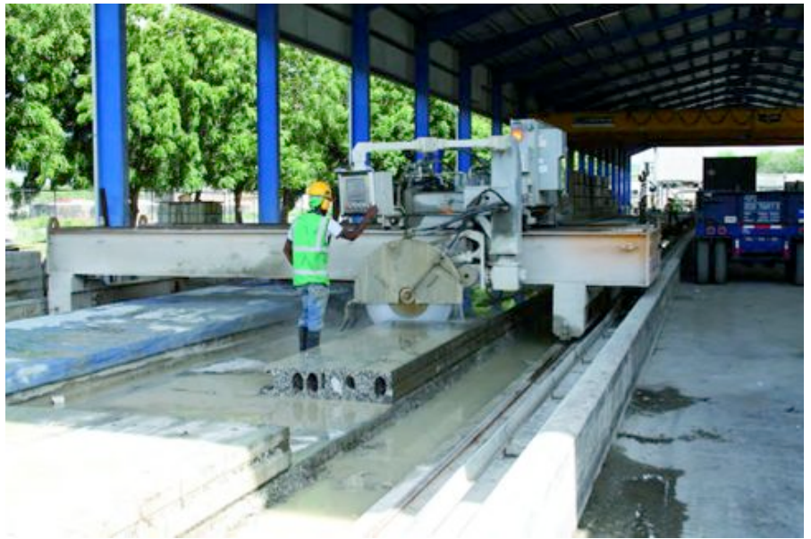
Fig.5: The hollow core slabs are cut to size after curing
