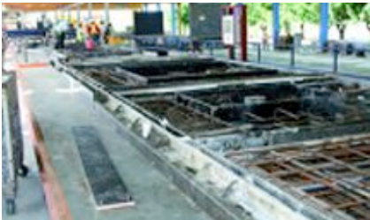
Fig. 12: Ratec magnets are used for moulding process that takes place on the upper level of the circulation plant.
